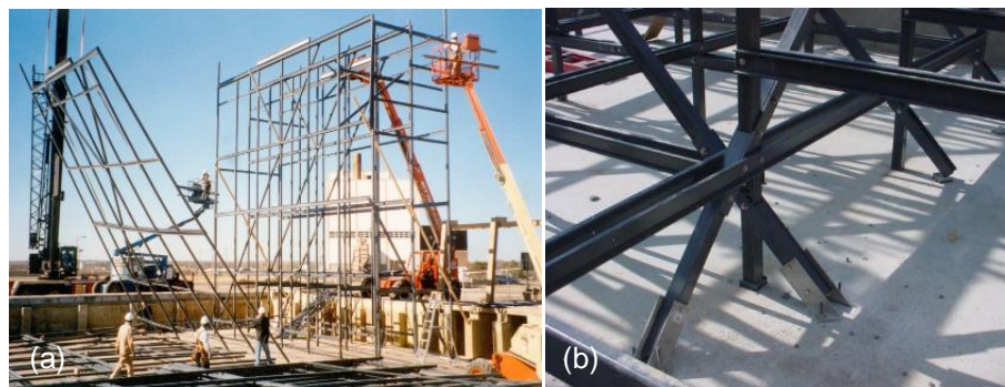
Figure 2.8. FRP stick-built cooling tower (image courtesy of Strongwell): (a) overview at erection; (b) close view of structural elements.
