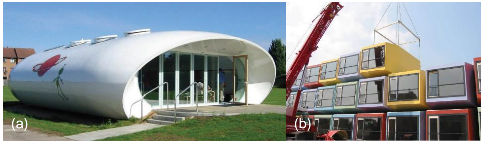
Figure 2.3. FRP modular buildings: (a) the Future Classroom (image courtesy of Altair HyperWorks) [29]; (b) the SpaceBox (image courtesy of Holland Composites) [30].
