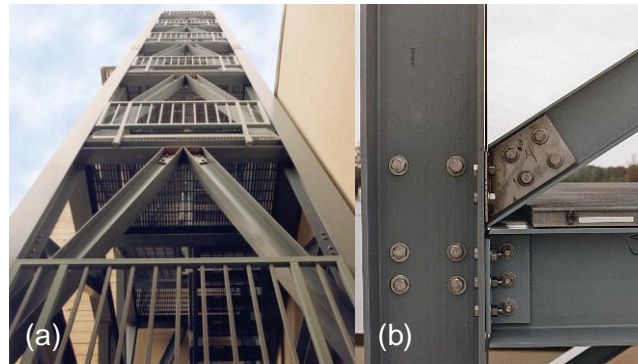
Figure 2.9. FRP stair-tower (image courtesy of Strongwell): (a) overview; (b) close view of connections.
