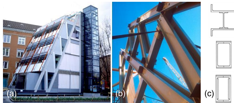
Figure 2.10. The Eyecatcher building: (a) overview (image courtesy of Fiberline A/S) [41]; (b) structural frame (with permission from Taylor & Francis) [42]; (c) built-up members [43].
