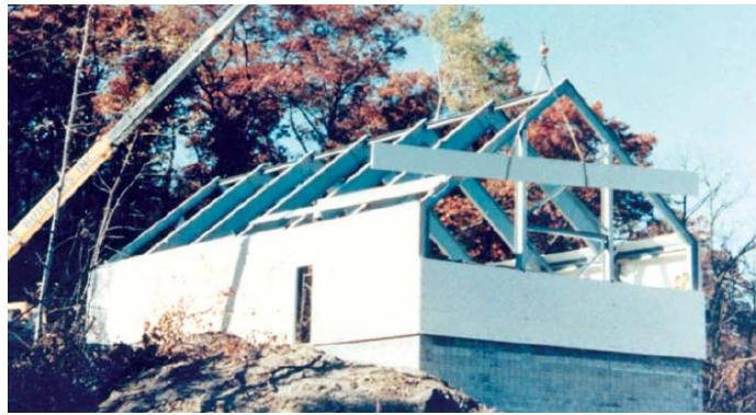
Figure 2.7. FRP portal frame structure for the testing of computer and electronic equipment (image courtesy of Strongwell) [38].
